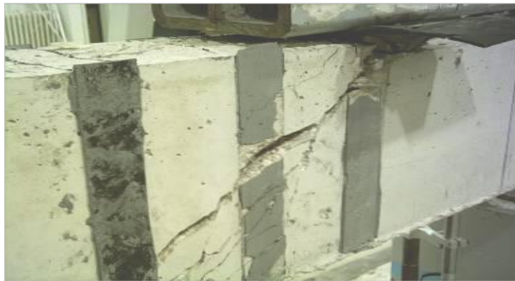
Fig. 18. Debonding and shear failures in group RS.
