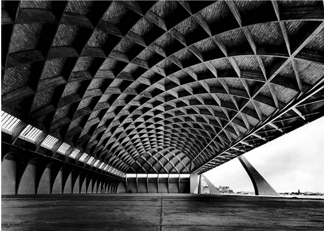
Figure 1.4: Pierre Luigi Nervi - Air hangar, built 1936
