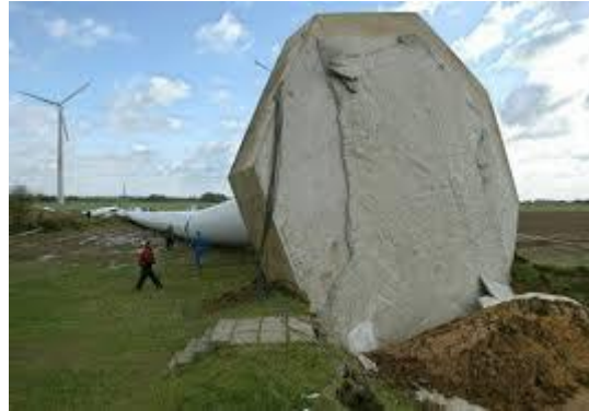
Figure 2 Stability considerations: overturning failure of a wind turbine foundation
