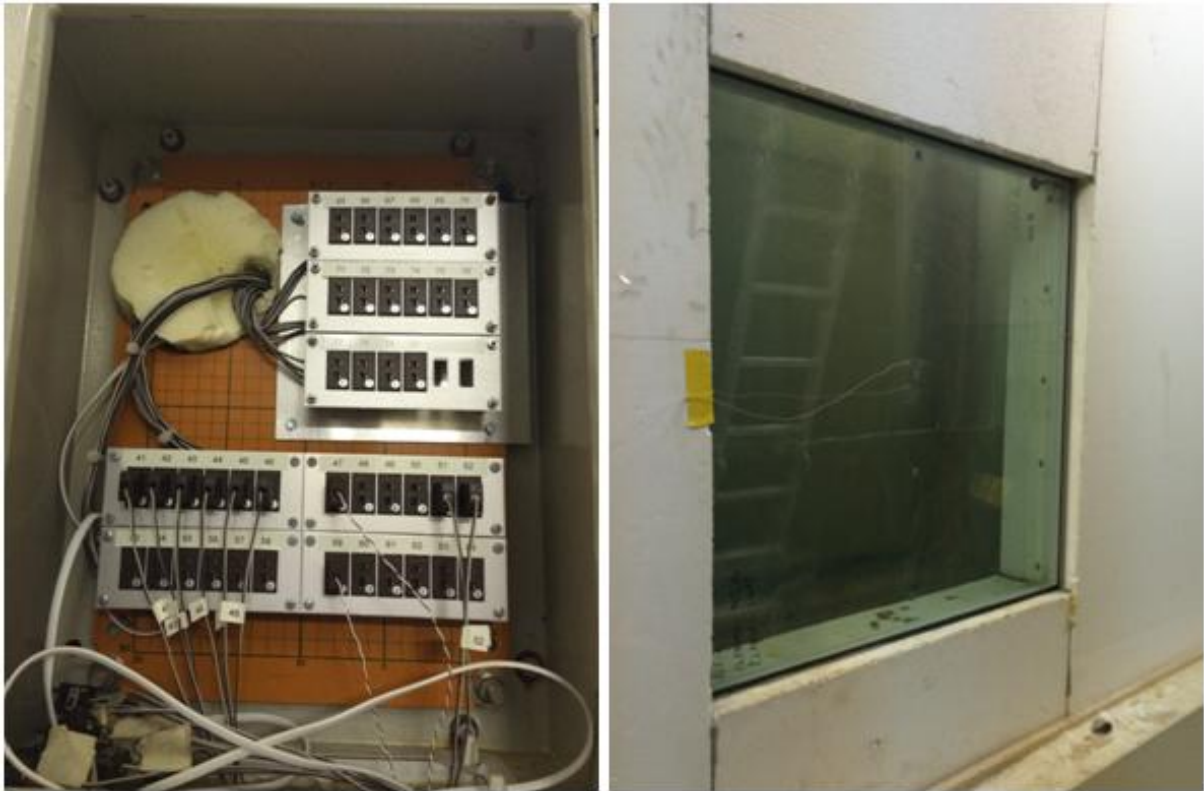
Figure 10. Left: Meter cabinet for thermocouple wires. Right: Installed IGU in Hotbox.
