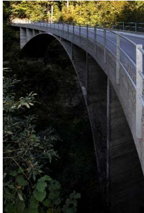
Picture 1. Schwandbach bridge by Robert Maillart 1933. (Source: Xpowa - Own work, CC BY-SA 3.0)
