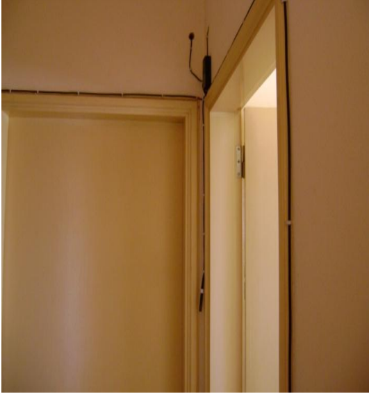
Figure 2.5(a) SHT75 temp. and RH sensor inside the flat
