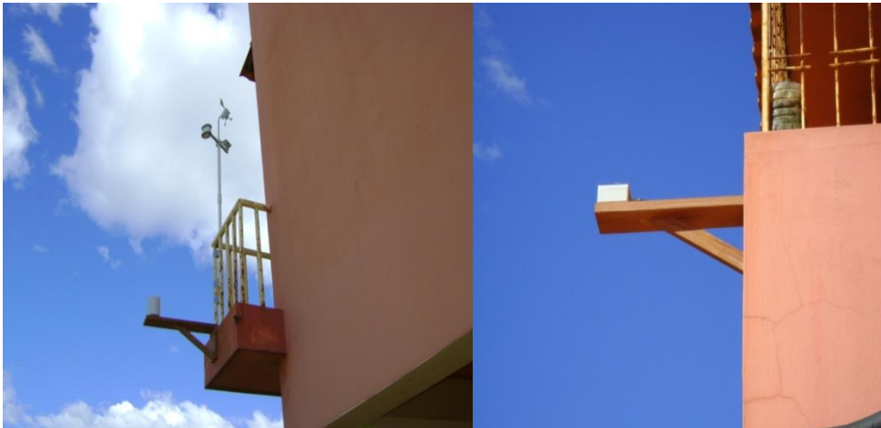
Figure 2.4 (a) Wind, temperature, humidity and rainfall sensors in the side of the building
