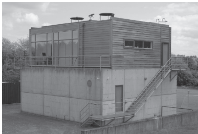
Figure 2.1 Picture of the Daylight Laboratory of the DBUR Institute showing the two experimental rooms, which are elevated from the ground (photo Jan Carl Westphall).
