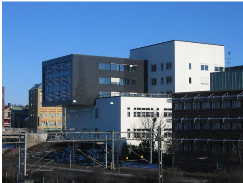
Figur 3.2 Tingshuset i Helsingborg [17]
