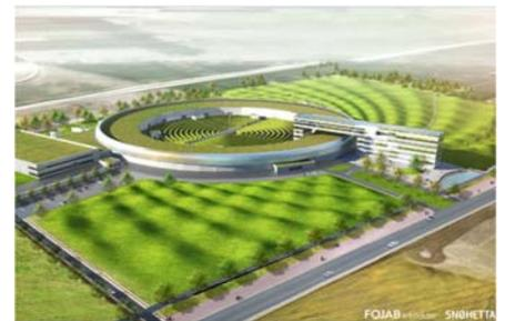
calculations imply that shaping the surrounding ground surface into a landscape of hills and valleys will reduce the incoming surface waves. Furthermore this is an aesthetically desirable solution, as the facility should serve the role as a landmark and a symbol of Lund as a technological capital.
