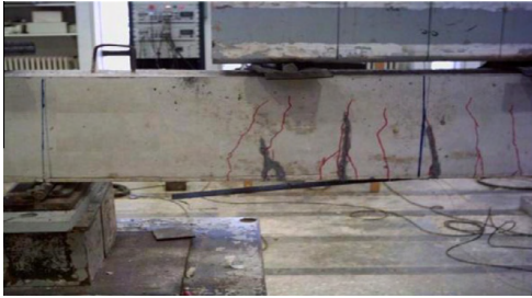
Fig. 15. Debonding failures in group RF.
