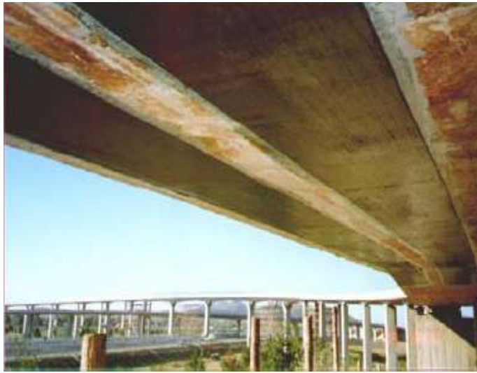
Figure 7: Flexural strengthening of a highway RC bridge slab in China, [10].
