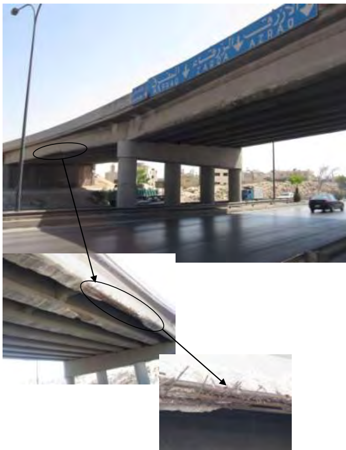
Figure 1: Bridge in the Al Zarqa-Jordan.
