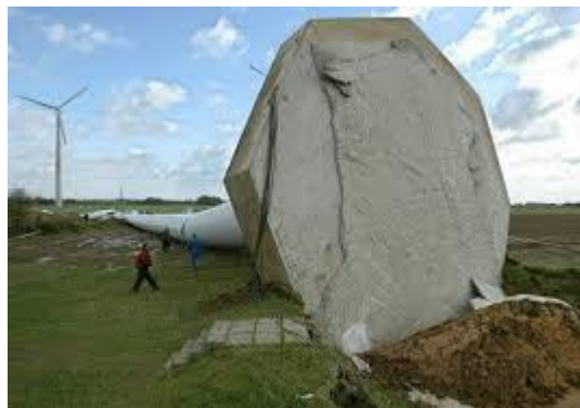
Figure 6 An overturning failure of a windmill [60].
