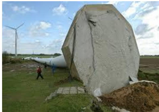
Figure 6 An overturning failure of a windmill [60].
