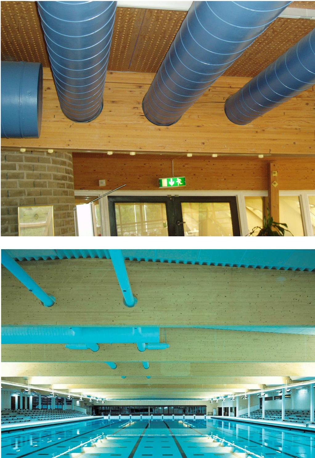
Figure 1.1: *Examples of constructions with glulam beams with holes. Top: Restaurant Ideon, Lund, Sweden. Bottom: Indoor swimming pool, Västerås, Sweden (with permission from Martinsons Trä AB).*
