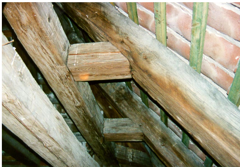
Picture 7.1 The beam supporting the rafter, seen from below.
