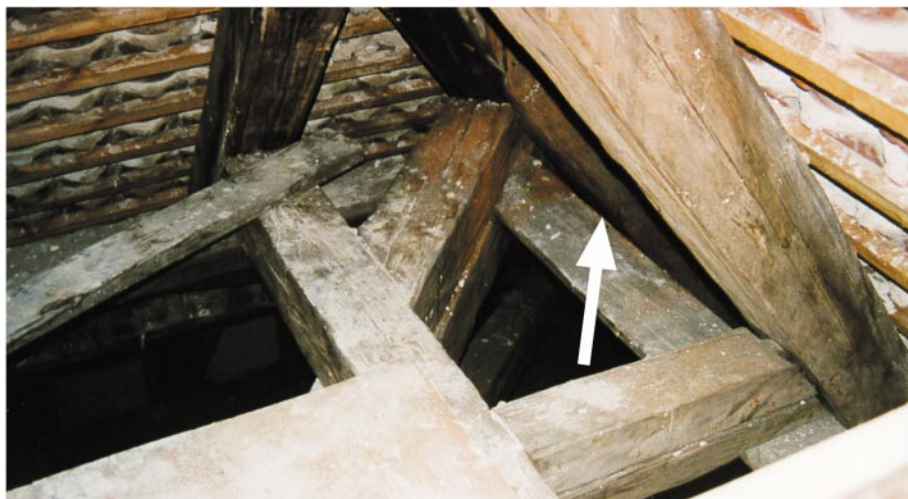
Picture 7.2 The picture shows the space between the rafters and the lying timberframe.
