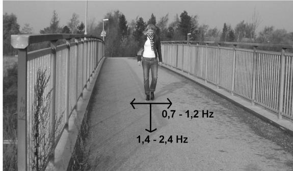
Figure 2.1: Vertical and horizontal forcing frequencies
