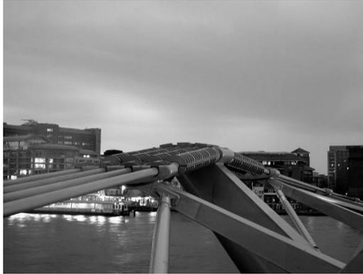
Figure 4.3: The cables are locked at each pier [36]
