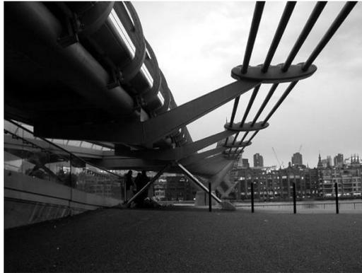
Figure 4.2: There are four cables on each side [36]
