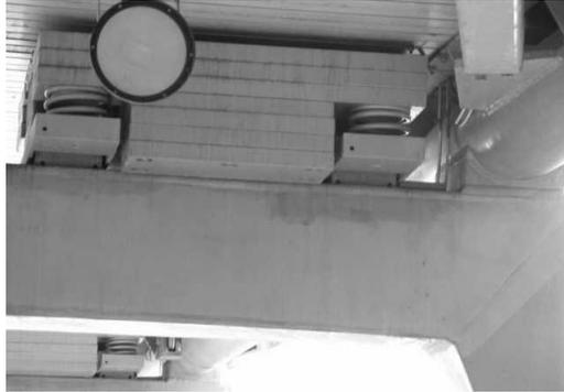
Figure 5.3: TMD beneath the deck
