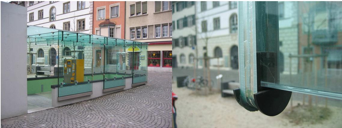
Figure 2.1: *The glass canopy over the stairwell to an underground carpark on the main square in Schaffhausen, Switzerland. The canopy is constructed with glass-beams supporting the roof. The right photograph shows a detail of the support of the beams with a spacer in a plastic material to distribute stresses*
