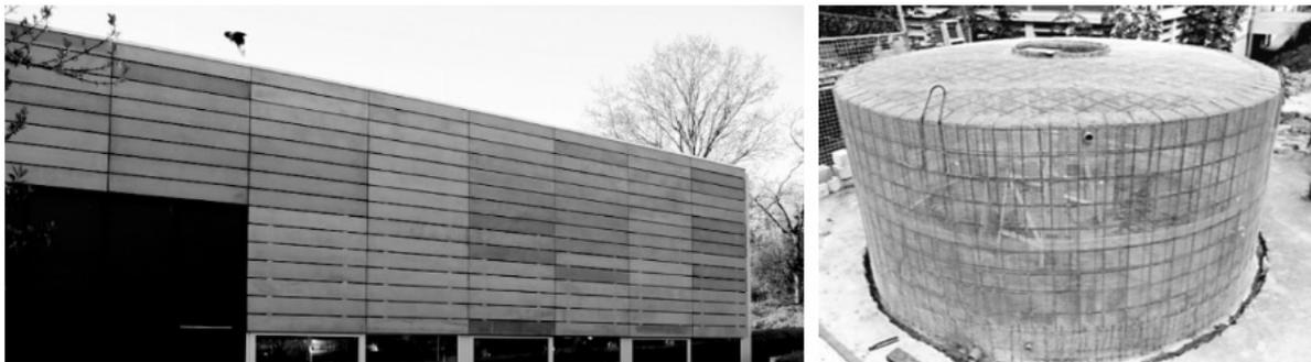
Figure 3.5: Left side, curtain wall construction the Institute of Structural Concrete, RWTH Aachen, Grosse (2007). Right side, ferrocement tank for rainwater collection, Arockiasamy et al. (2009).
