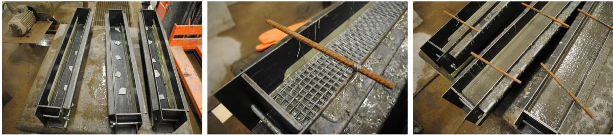
Figure 4.8: Anchored steel reinforcement in formwork.
