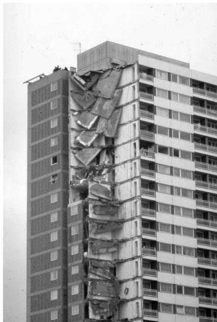
Figure 3.8: Progressive collapse of Ronan Point building [51].
