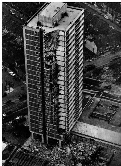
**Figure 1.1:** Ronan Point after an explosion in 1968, retrieved from [1].
