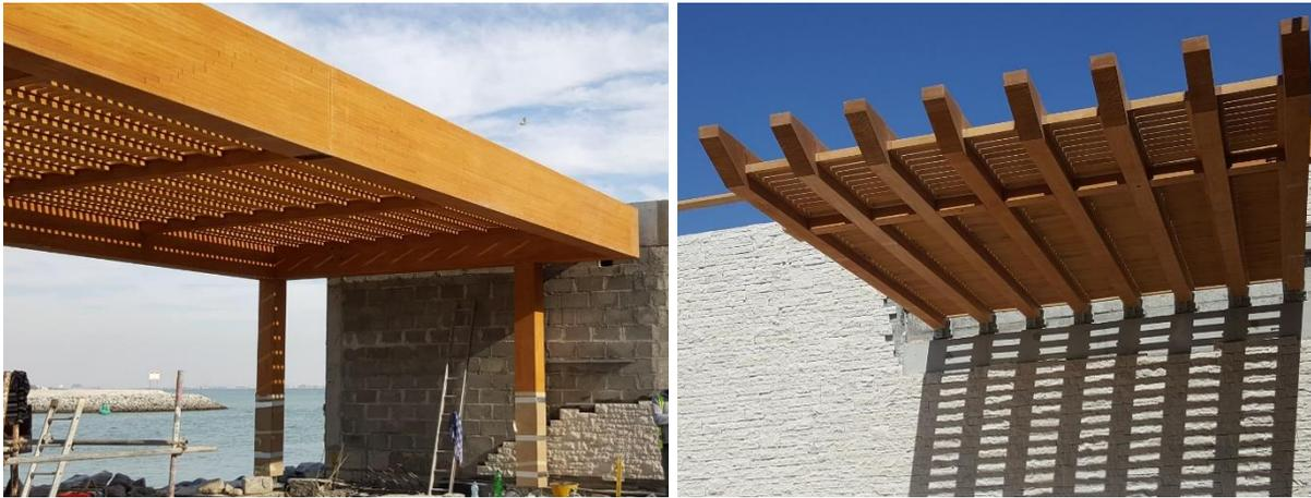
Figure 37. Examples of use in outdoor structures. Left: Portal frames with post/beam moment resistant connections. Right: Rafters with moment-resistant connections fixed on a wall.
