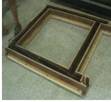
Figure. 4.1 Form work and laying reinforcements for beam and column elements
